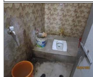
Photo of the sanitary facilities toilet.JPG
